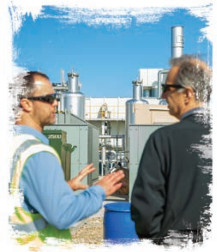
Director of the Department of Waste & Renewables John Welch (left) and County Executive Joe Parisi (right) overlook the recently completed RNG facility in Dane County.
