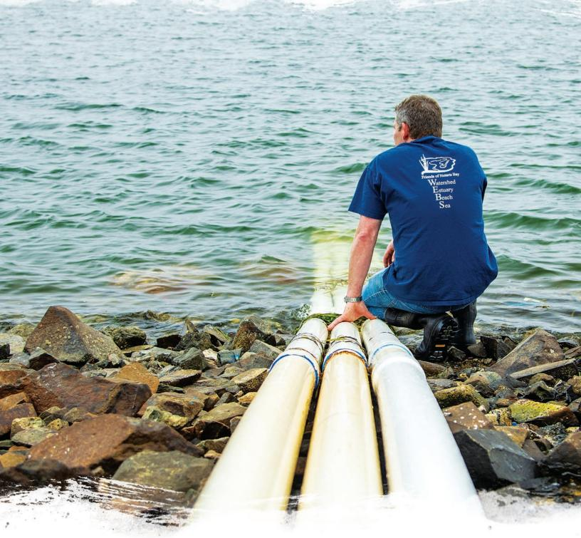
Alan Barton, manager of Whiskey Creek Shellfish Hatchery, overlooking Netarts Bay. The pipes draw water from the bay into the hatchery for filling the tanks. In the past, the water was used directly from the bay. Today, the hatchery has to buffer all of the water for use. Credit: Impact Media Lab / AAAS
